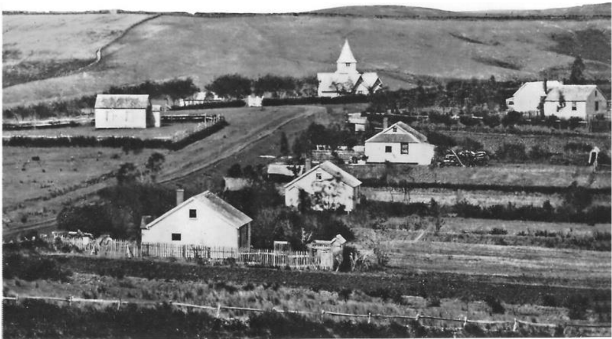
Figure 8. Picton Street Howick looking East with All Saints Church in background and Fencible cottages in foreground; circa 1860; Image kindly provided by Howick Historic Village 1013 .
