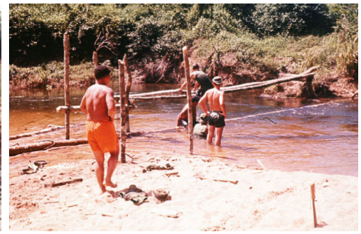
2NZR-10-Platoon-D-Company-081 | Building bridge between camp and L-Z north Malaya close to Thai border early 1961. Image taken during Malayan Emergency 1959-1960. © Peter Gallacher.
