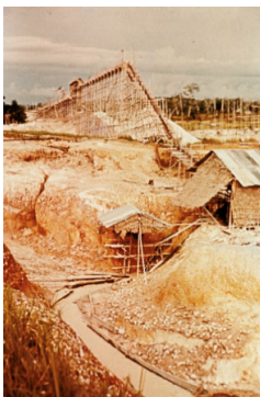
2NZR-10-Platoon-D-Company-227 | Landscape showing construction. Image taken during Malayan Emergency 1959-1960. © Peter Gallacher.
