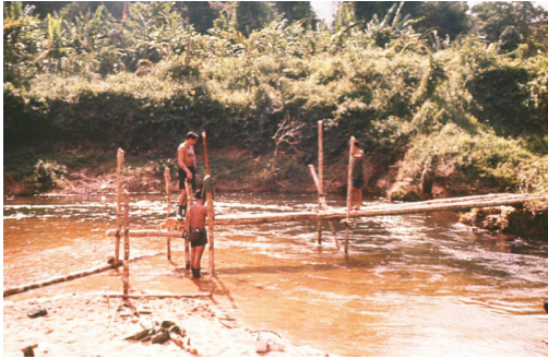
2NZR-10-Platoon-D-Company-082 | Bridge under construction. What part next?. Image taken during Malayan Emergency 1959-1960. © Peter Gallacher.
