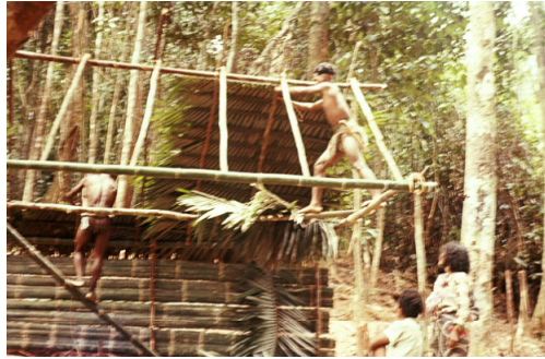
2NZR-10-Platoon-D-Company-219 | Orang Asli putting atap roof on house. Image taken during Malayan Emergency 1959-1960. © Peter Gallacher.
